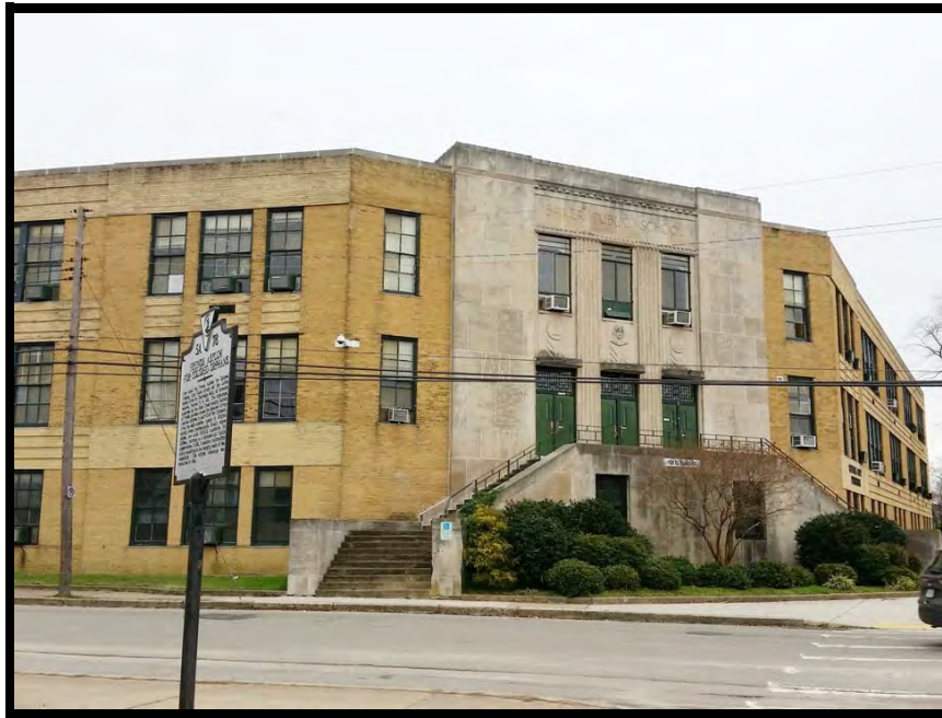
View of site from the north
