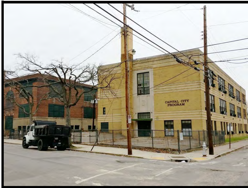
View of site from the northeast
