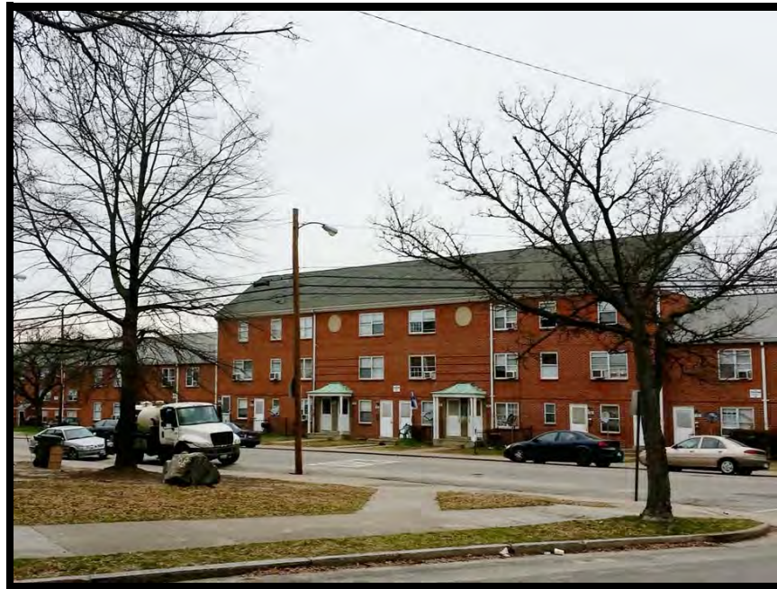
Northwest view from site
