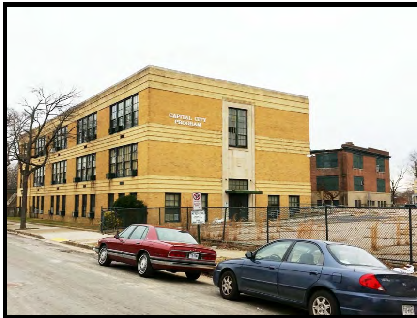
View of site from the west
