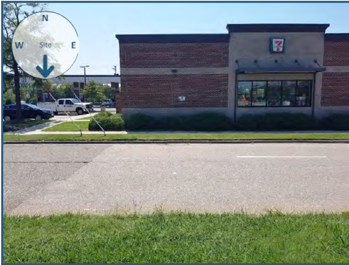
South view from site
