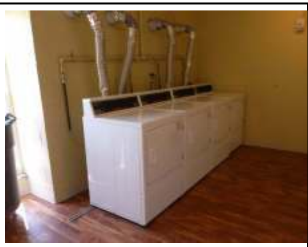
View of typical laundry room
