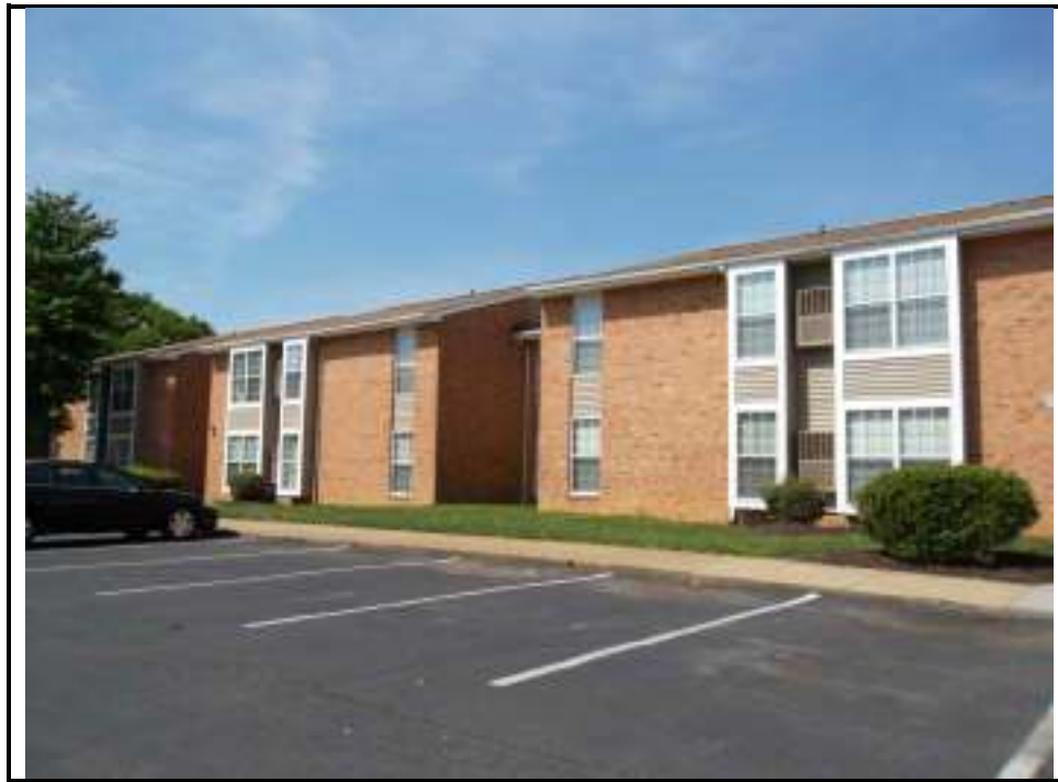
Exterior view of subject buildings facing east
