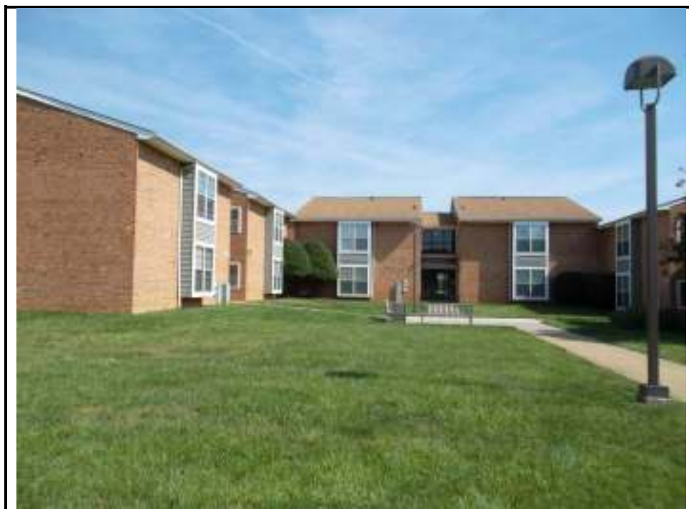
Exterior view of subject buildings facing north
