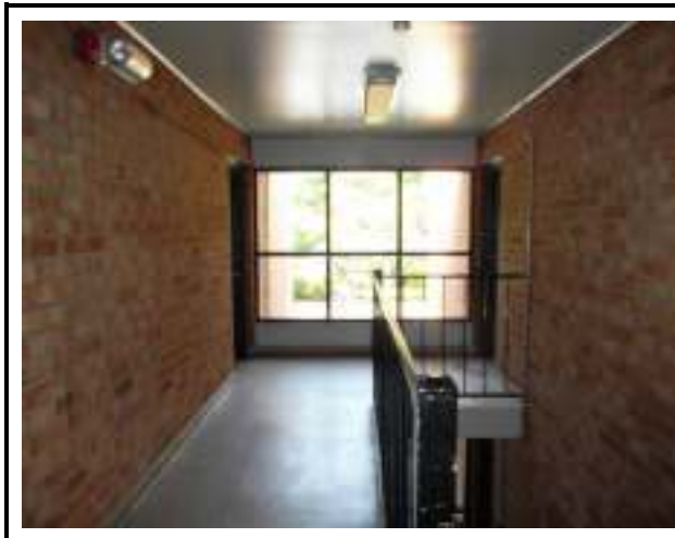
View of typical interior stairwell
