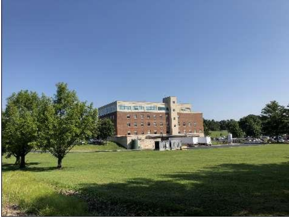
View to the North
