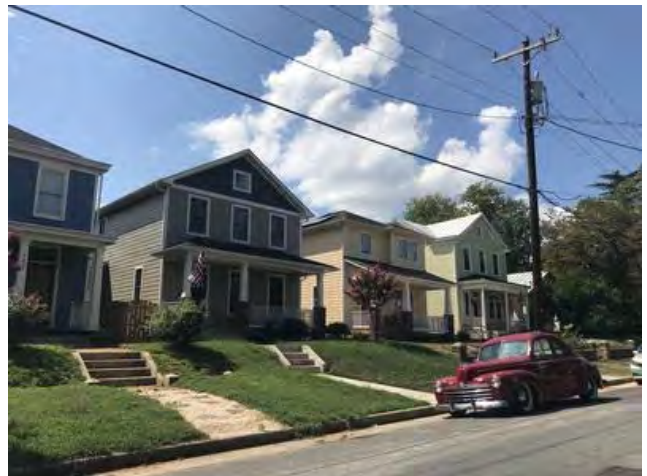
Typical single-family homes in Subject neighborhood
