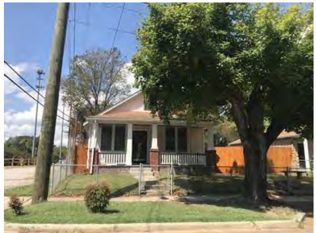
Typical single-family homes in Subject neighborhood
