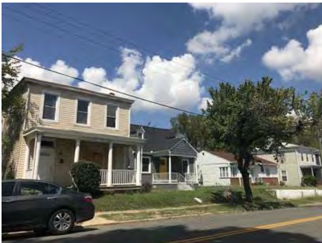
Typical single-family homes in Subject neighborhood
