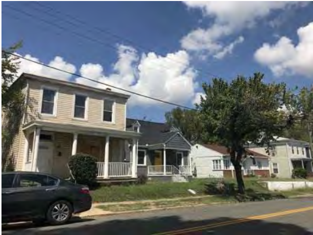
Typical single-family homes in Subject neighborhood
