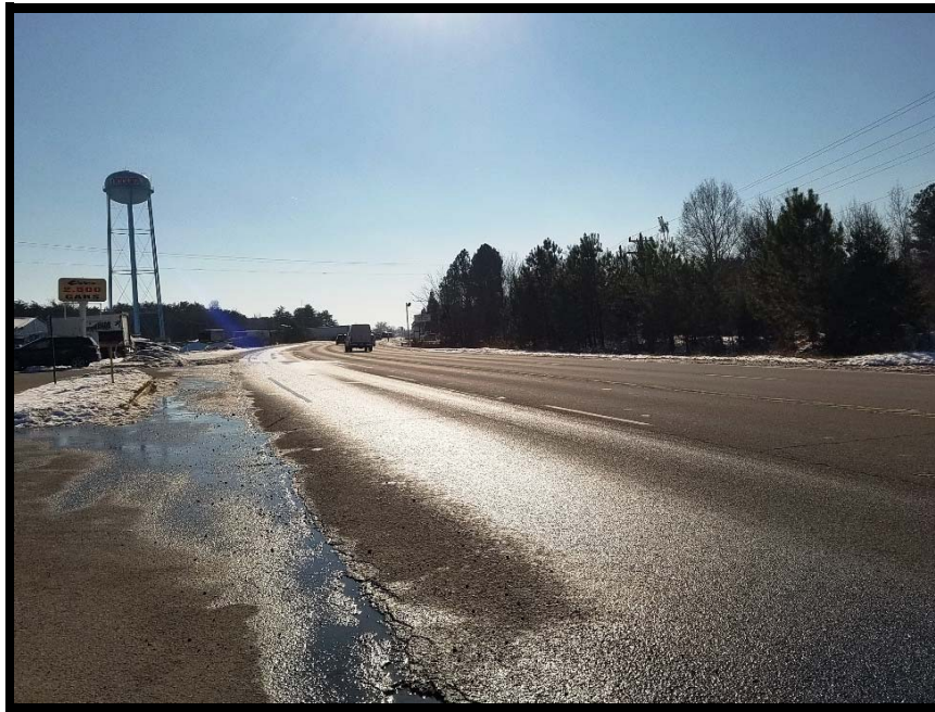
Streetscape: South view of U.S. Highway 1/Jefferson Davis Highway
