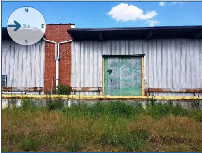
View of site from the west
