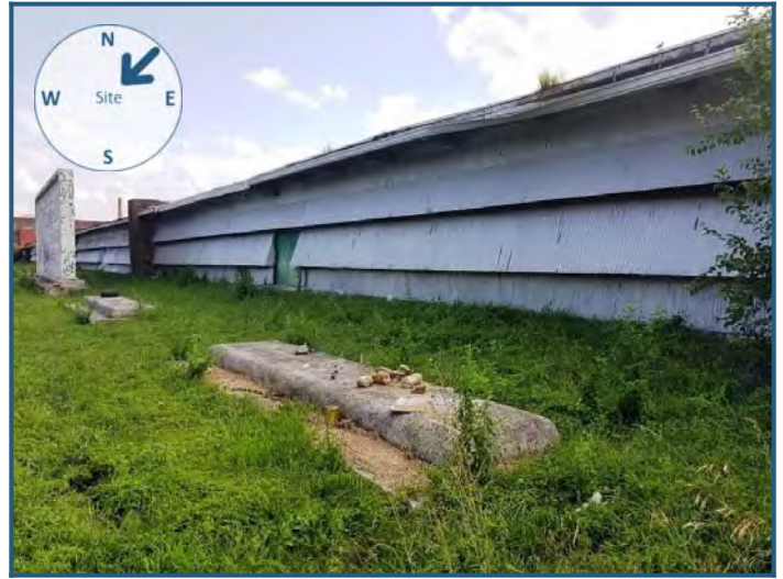
View of site from the northeast
