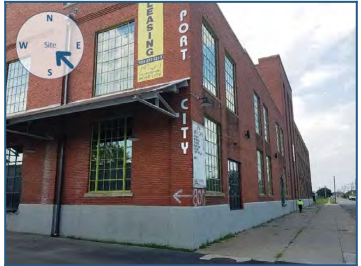
View of site from the southeast
