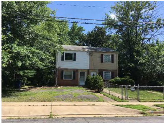
Existing duplex structures on site at Biscayne Dr. and Glendale Terrace (NE) to rear of brick apartment structure
