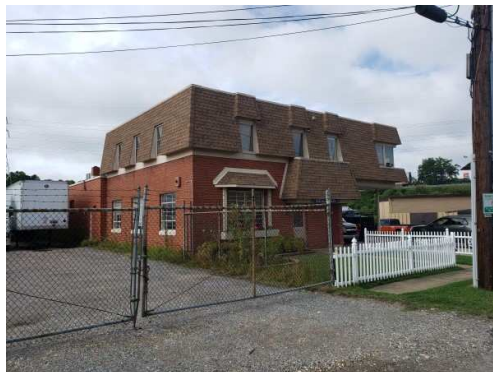
Keheller HVAC building north of site.
