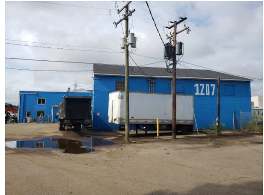
Existing structure onsite (to be demolished).
