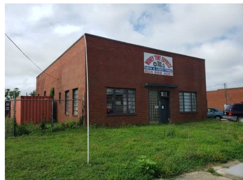
Money Tire Express building north of site.
