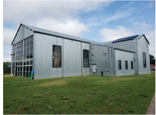
Dovetail Construction east of site.
