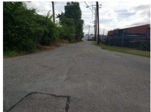
Sledd St south of site.
