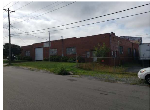
Virginia Cabinetry building north of site.
