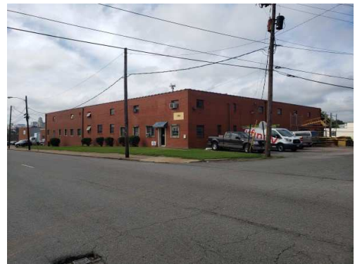
Multi-tenant two-story flex building south of site.
