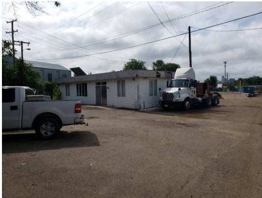
Existing structure onsite (to be demolished).
