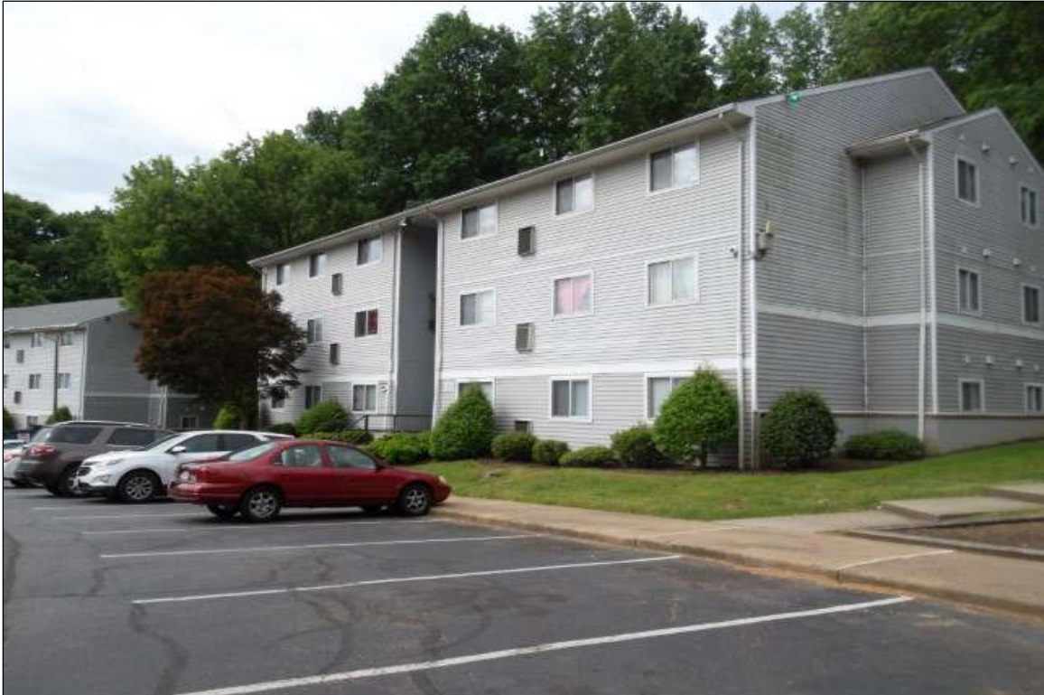
View of typical subject building facing southwest
