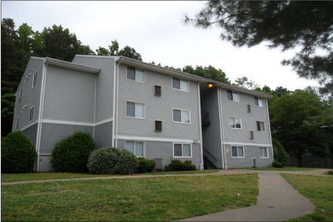
Rear view of typical subject building facing north
