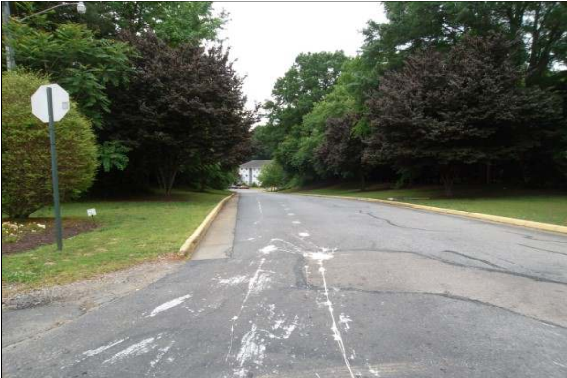
Walmsey Boulevard facing west
