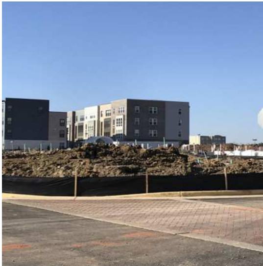
Pulte Condominiums under construction west of subject
