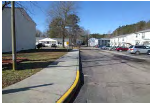
Looking West from Entrance
