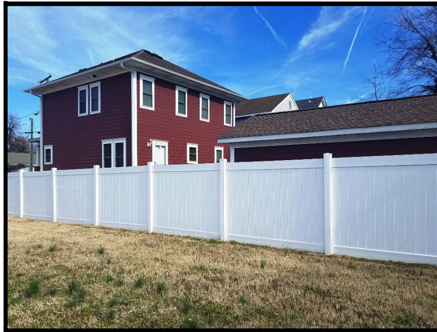
Northeast view from site
