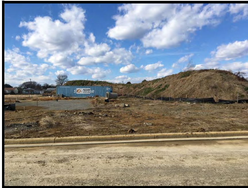
View of site from the southeast
