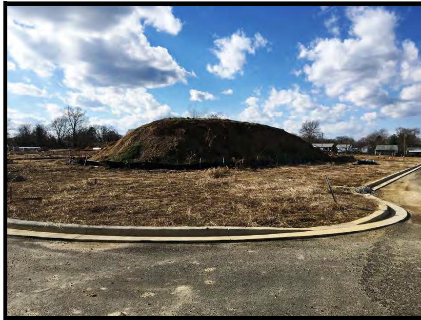
View of site from the east
