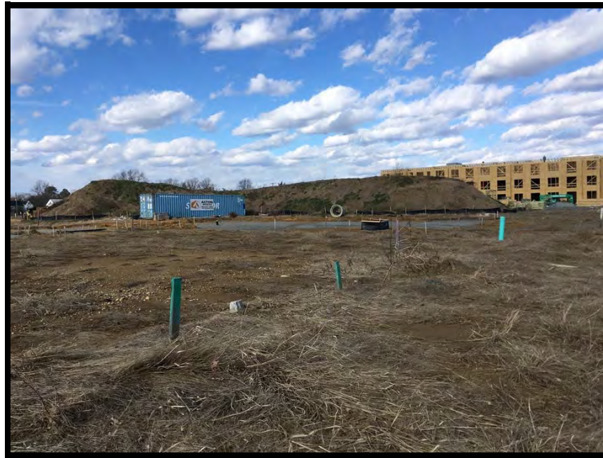
View of site from the south
