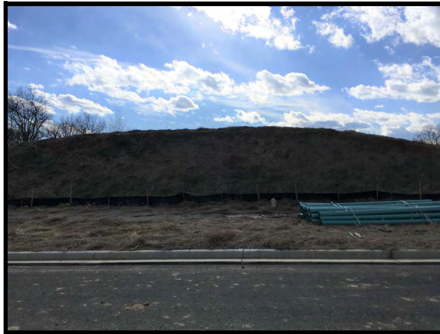
View of site from the northeast
