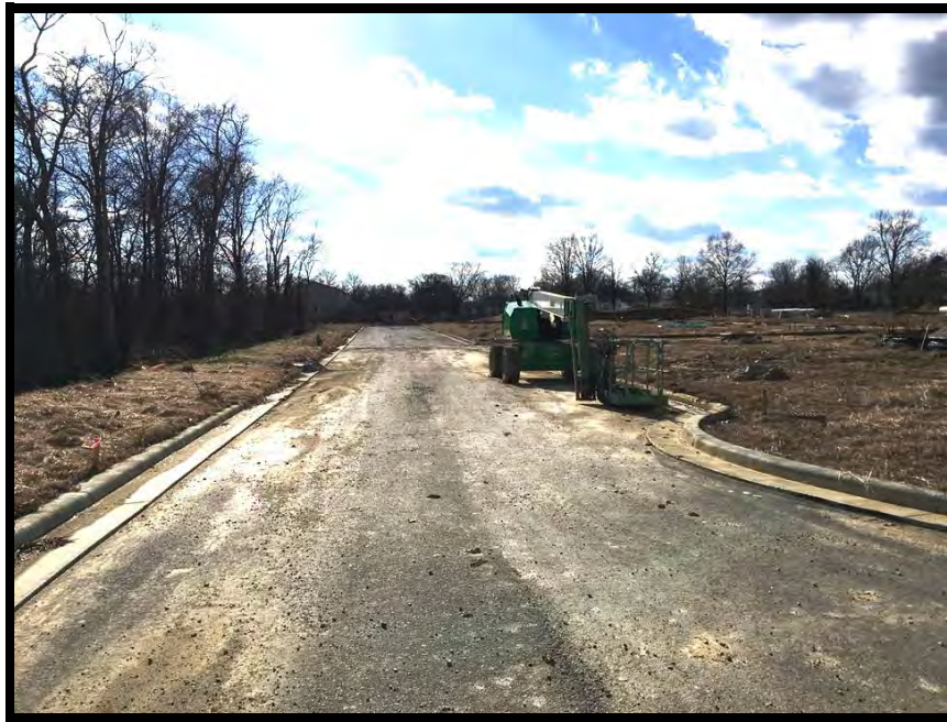
Streetscape - Southwest view
