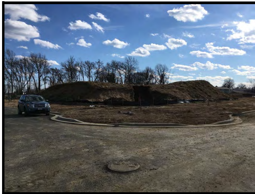
View of site from the north
