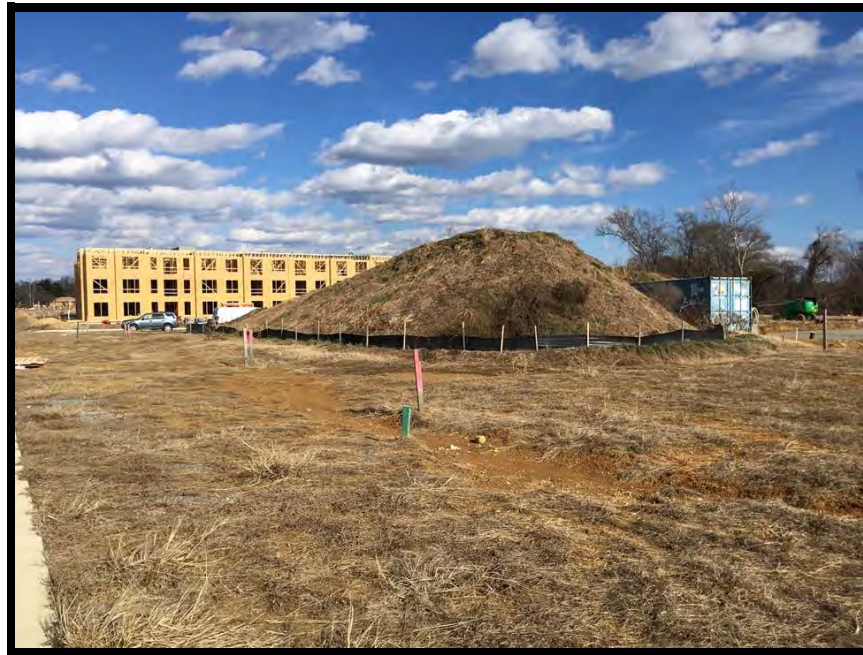
View of site from the west
