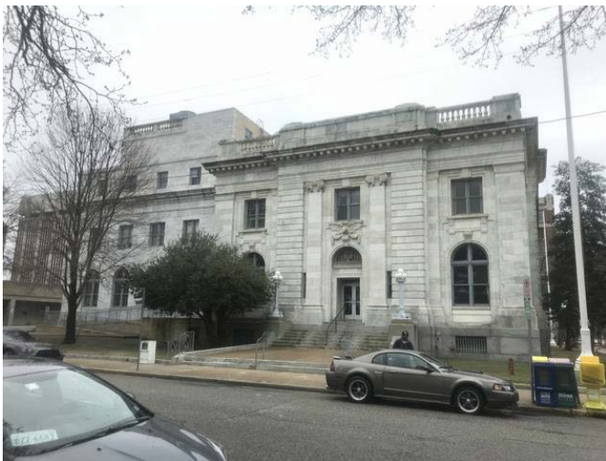
Post office south of the Subject site
