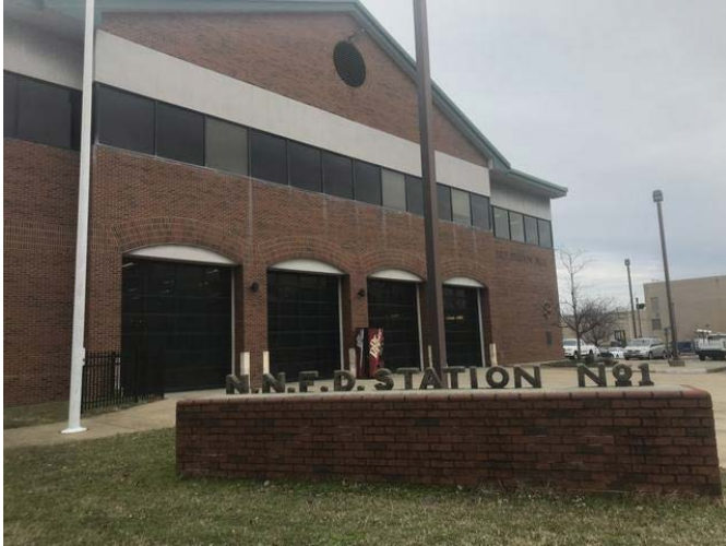
Fire station west of the Subject site
