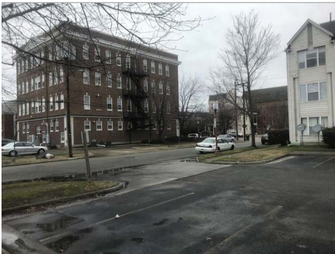
Subject site looking northeast
