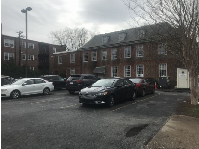
View west from the Subject site
