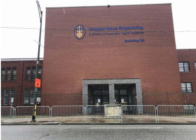
Newport News Shipbuilding west of the Subject site
