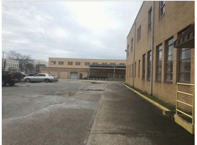
Commercial use south of the Subject site
