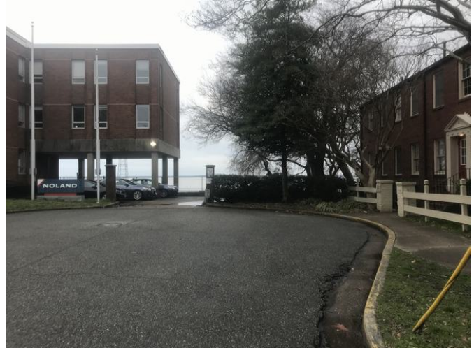
View west from the Subject site
