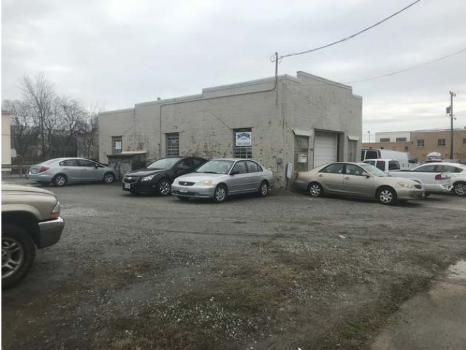
Garage north of the Subject site
