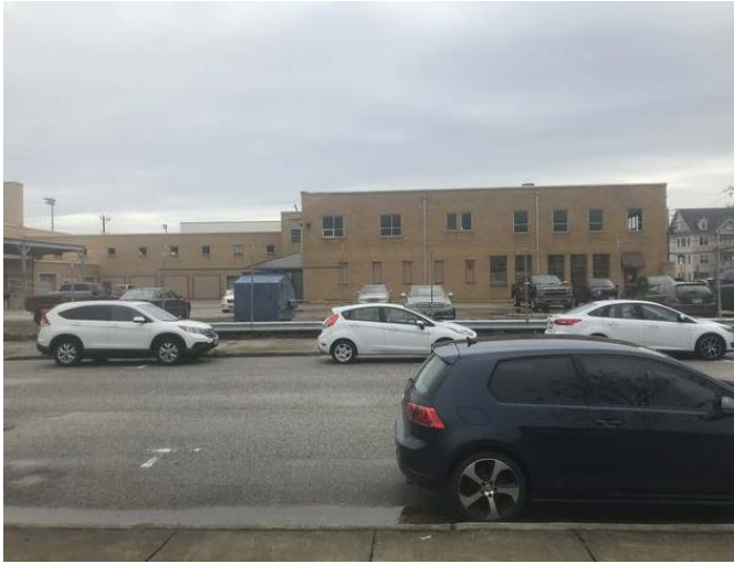
Commercial use south of the Subject site
