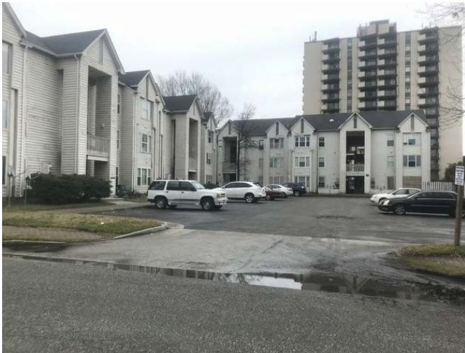
Subject site looking south
