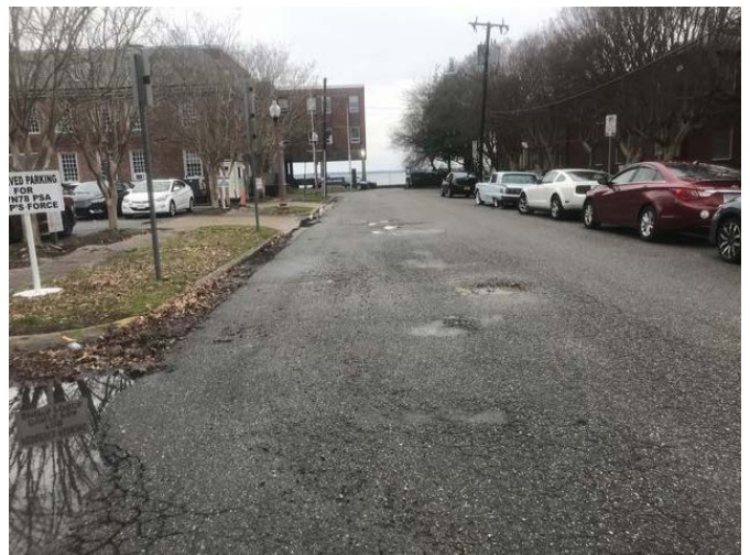
View looking west on 29th Street
