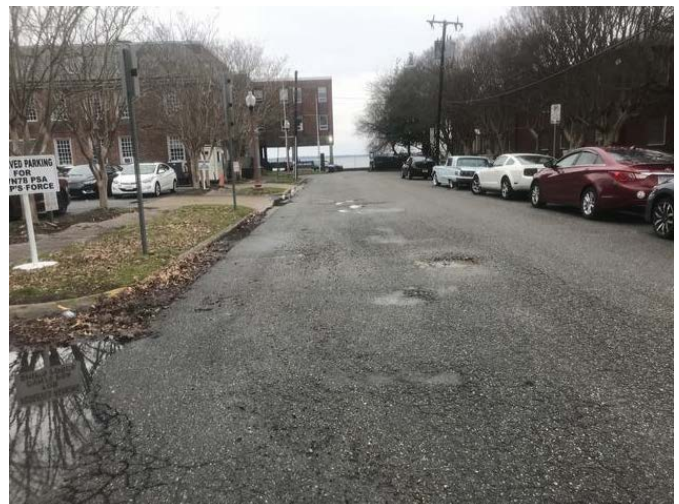
View looking west on 29 th Street
