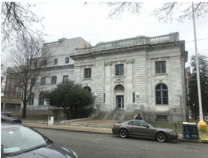
Post office south of the Subject site
