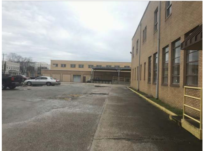
Commercial use south of the Subject site
