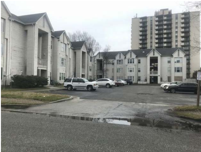
Subject site looking south
