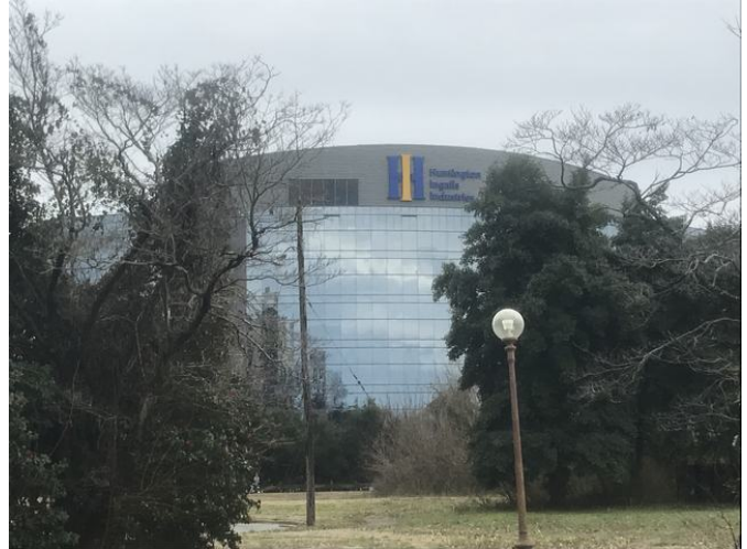
Office building/shipbuilding facility south of the Subject site
