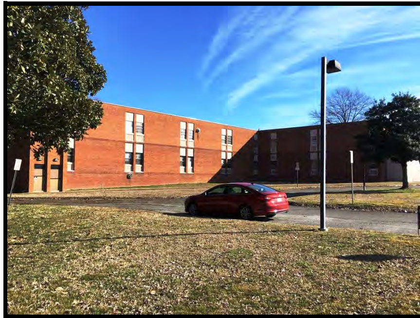
View of site from the southwest
