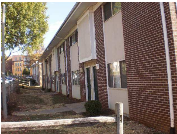
View of existing buildings in interior of site
