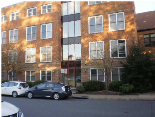
Norcross Station new construction building
