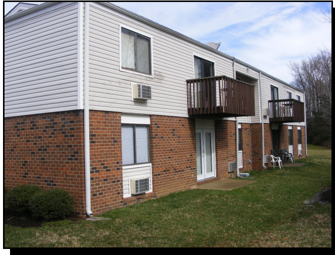
Typical units - rear view
