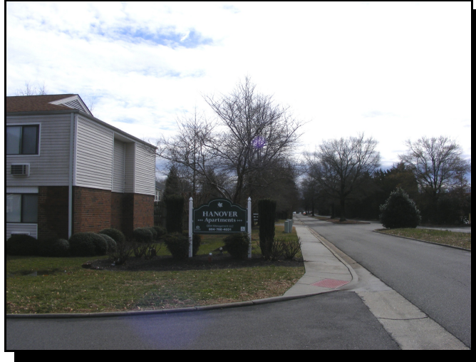
View north on N.Cottage Green Dr., at entrance
