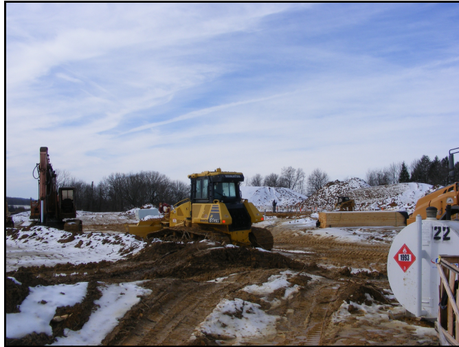
Ongoing construction of project
