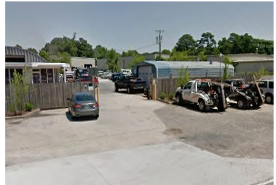
Commercial facility northeast of subject site along Curlew Drive
