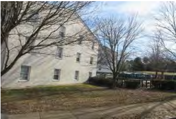
Looking East From Entrance
