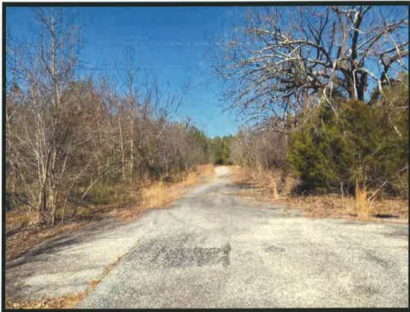
Streetscape - North view along Krouse Street
