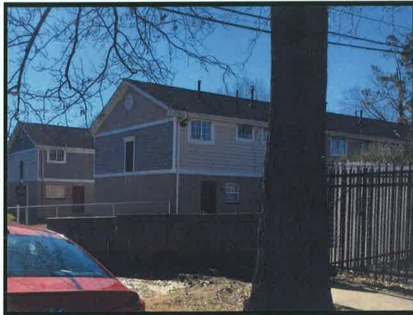
Southwest view from site
