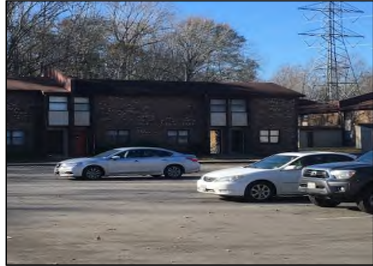
Subject building facing west.
