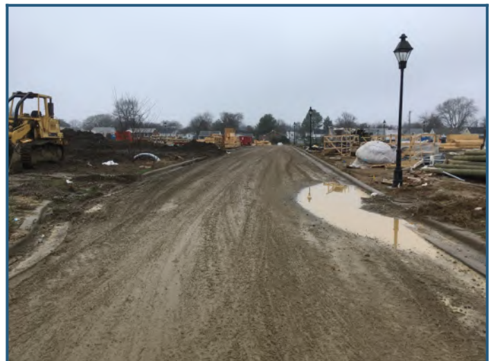
Streetscape: Southwest view
