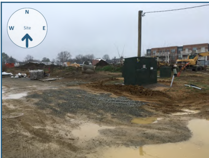
View of site from the south
