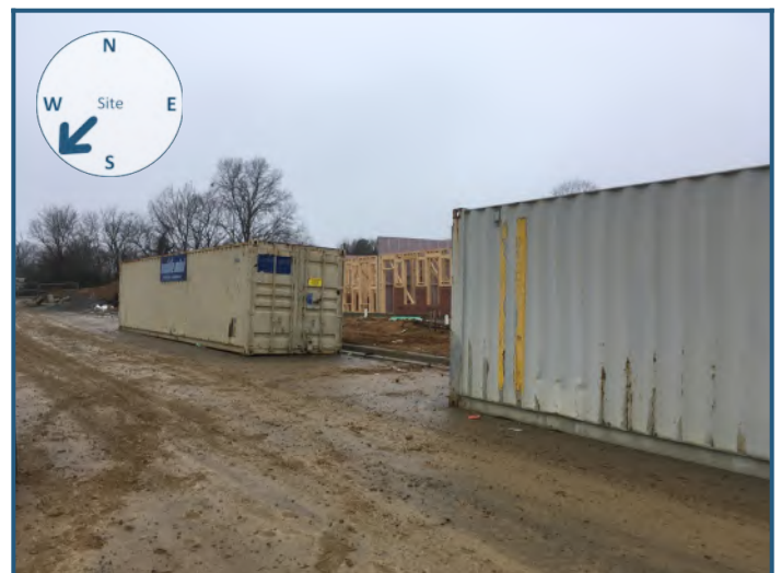
Southwest view from site
