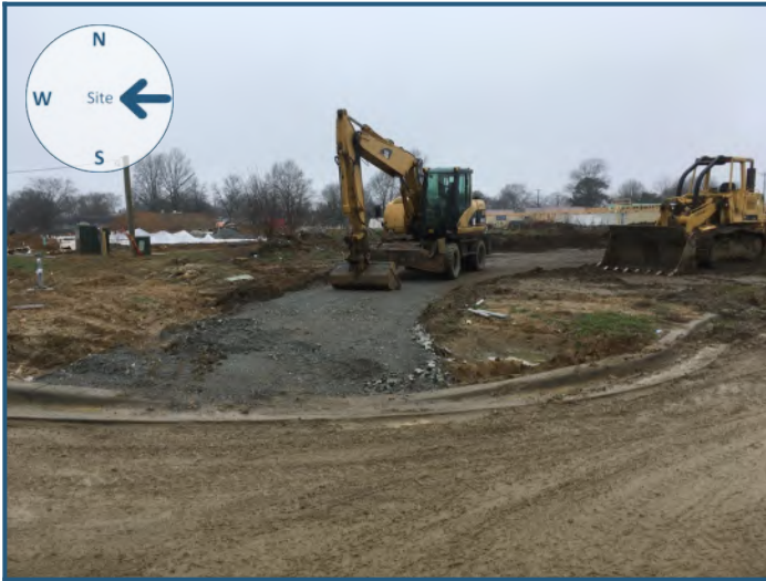
View of site from the east
