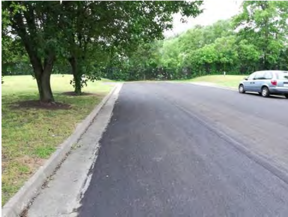
View of New Hunter Road – To the North
