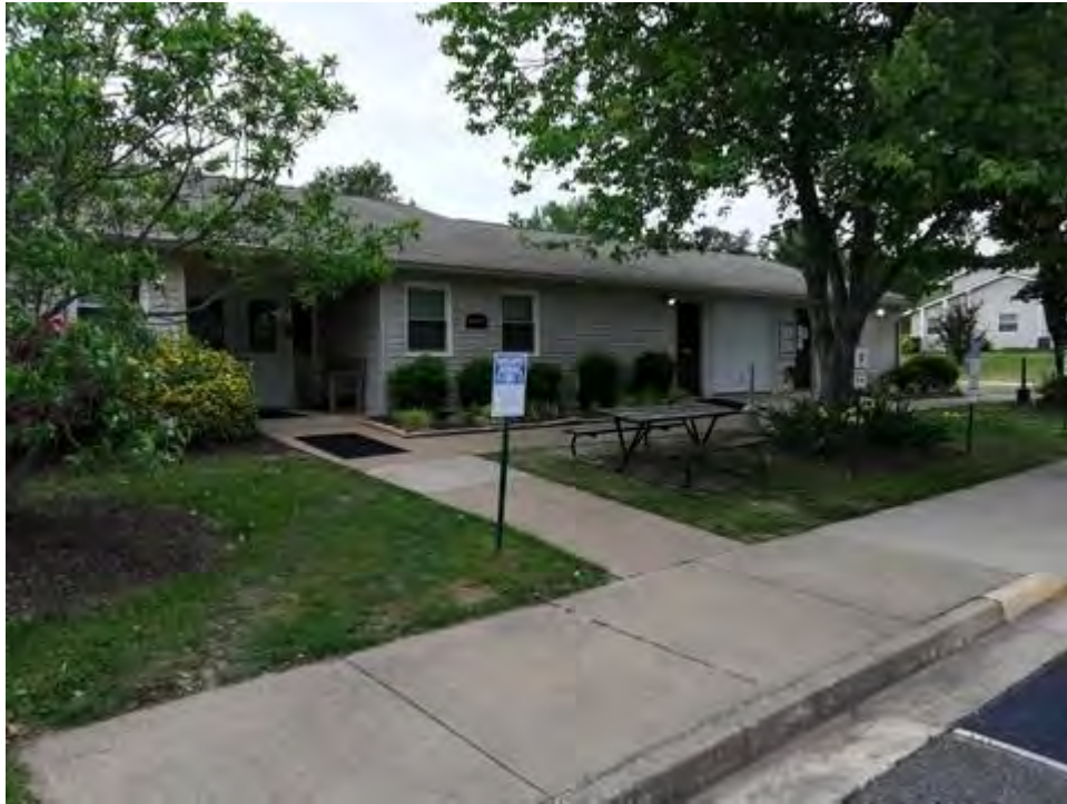
View of Accessory Building – Exterior
