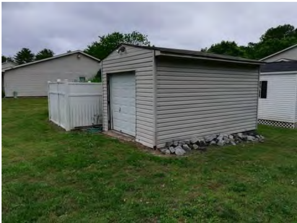
View of Maintenance Storage Shed
