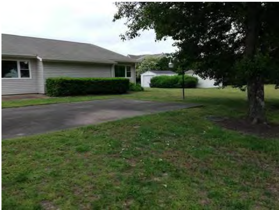
View of Former Shuffleboard Court (Not In Use)
