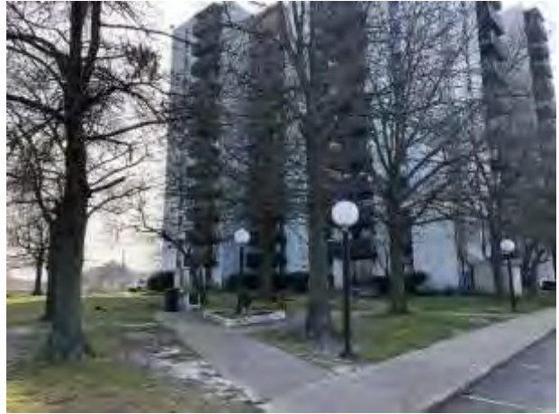
Subject building from side yard
