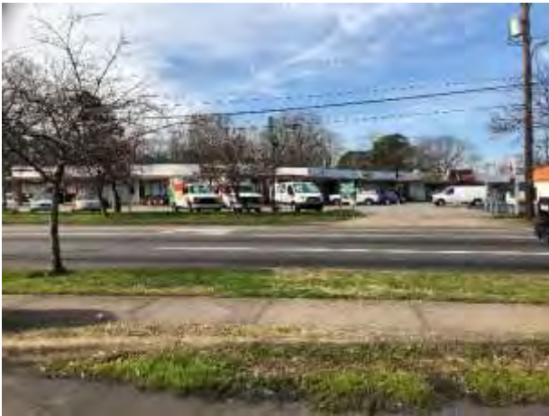
Strip center in average condition on Tidewater
