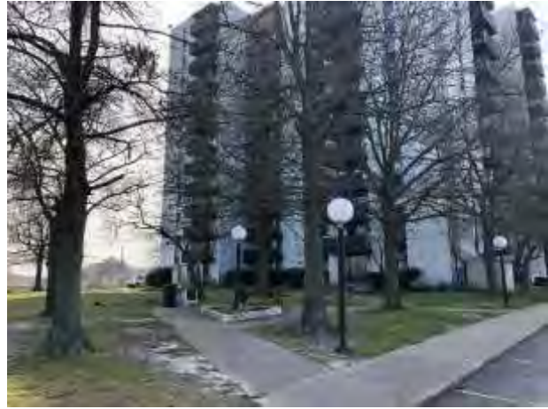
Subject building from side yard
