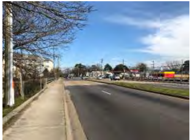
View looking north on Tidewater
