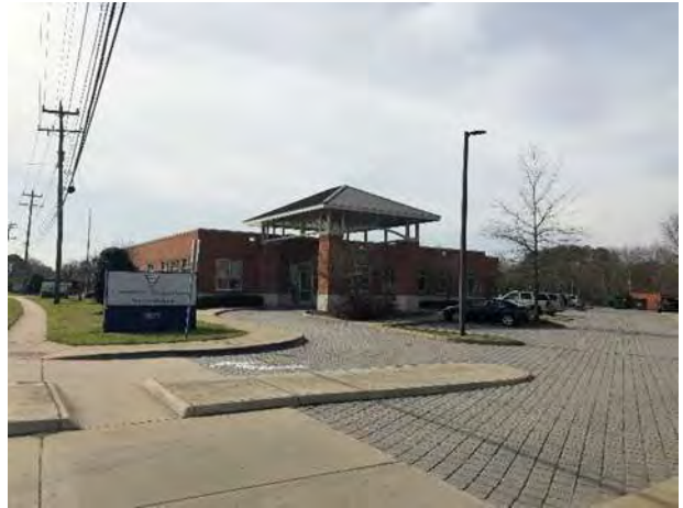
Health center next to Subject
