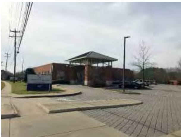
Health center next to Subject
