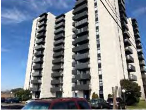
Subject building from entry drive
