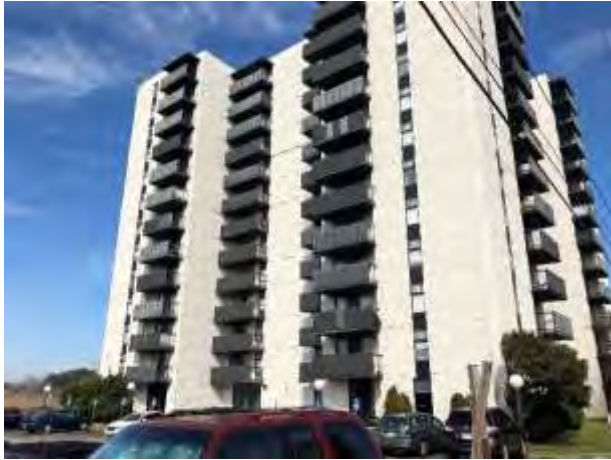
Subject building from entry drive
