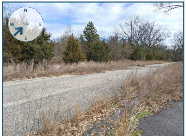
View of site from the southwest
