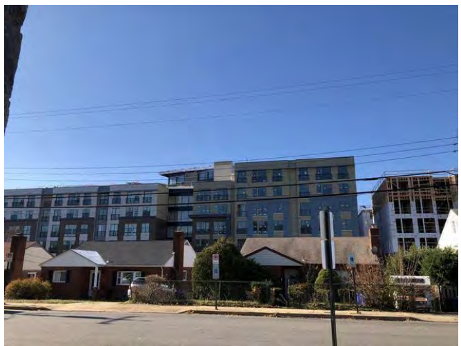
Typical single-family with The Trove, market rate housing development under construction and located directly northwest of the Subject
