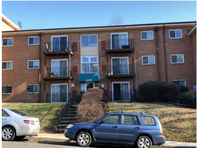
Subject site (improvements to be demolished)
