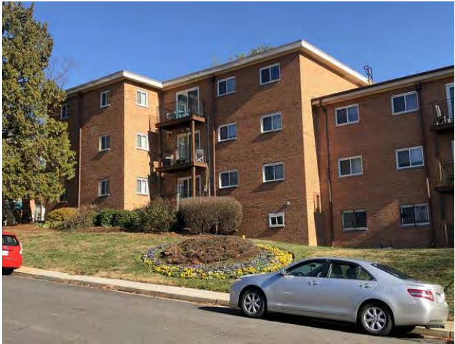
Subject site (improvements to be demolished)
