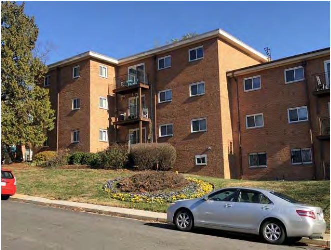
Subject site (improvements to be demolished)
