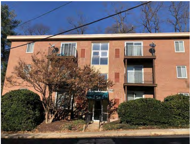
Subject site (improvements to be demolished)
