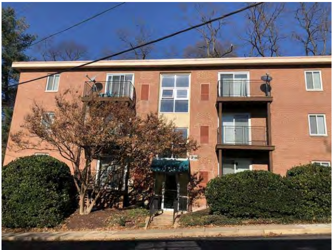
Subject site (improvements to be demolished)
