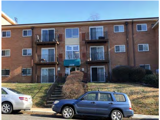
Subject site (improvements to be demolished)
