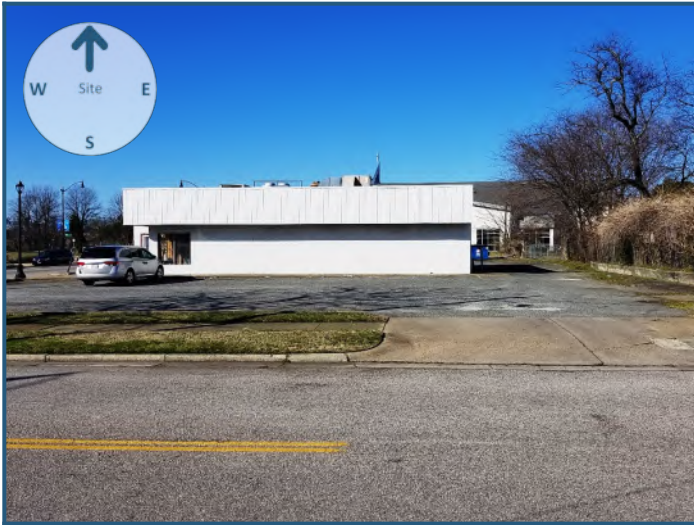
North view from site
