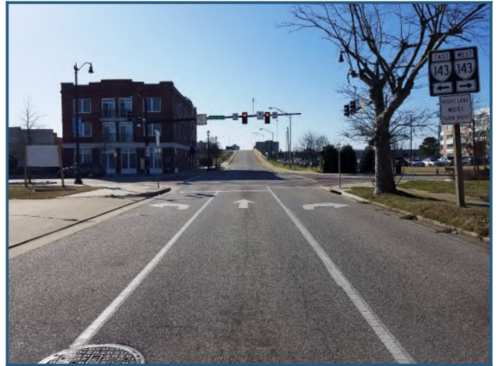
Streetscape: West view of 28th Street
