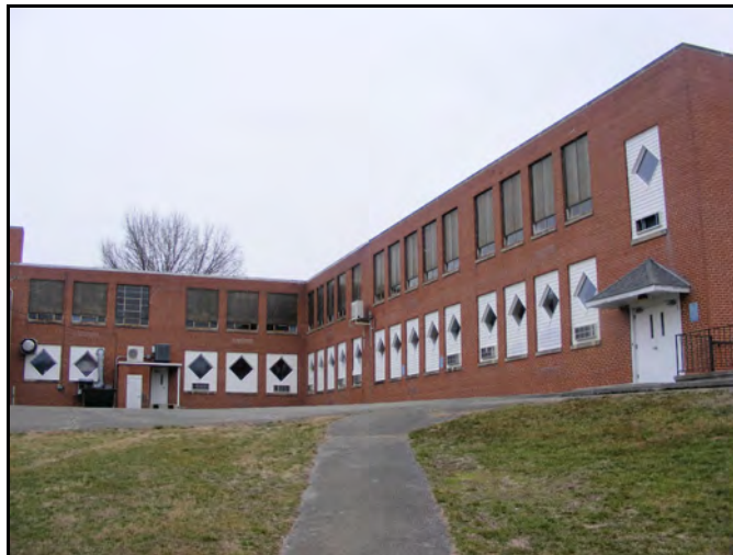
View of the rear of the property
