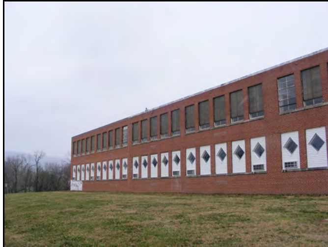
View of the side of the property
