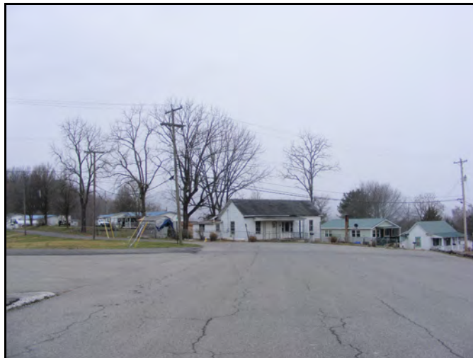
View towards Ward Lane at front of property
