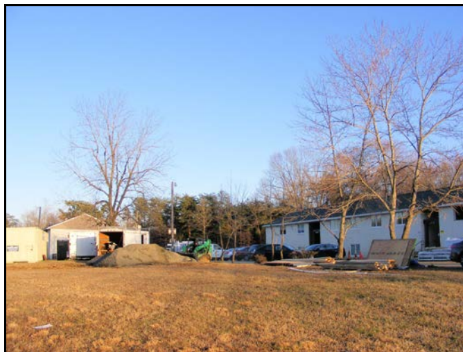
Ongoing rehabilitation at East Gate Village
