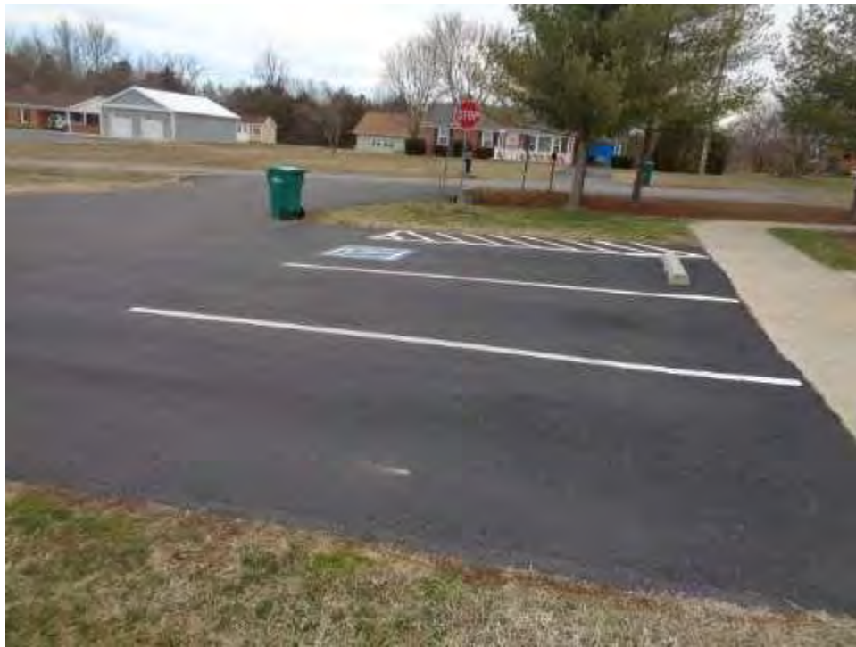
View of Parking
