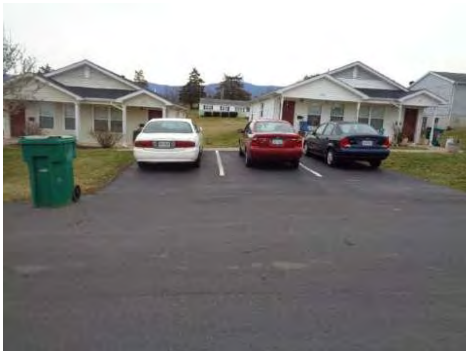
View of Parking
