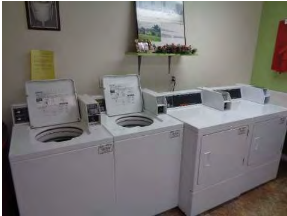
View of Laundry Facility
