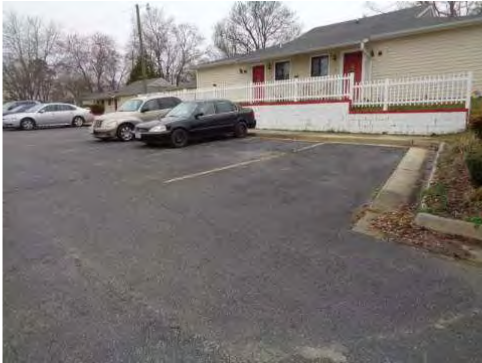
View of Parking
