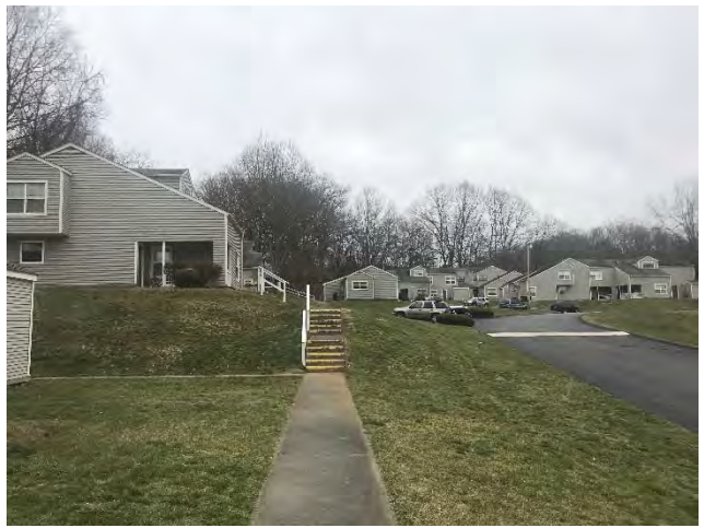
SUBJECT PROPERTY AND TYPICAL WALKWAY
