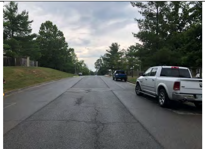
VIEW NORTH ON FAIRFAX STREET
