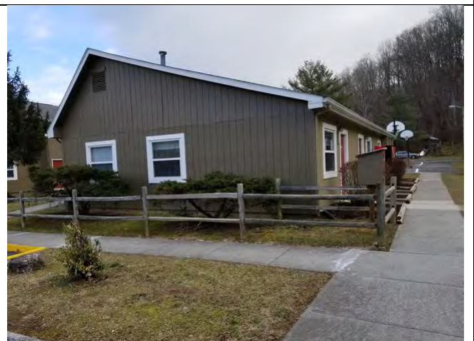
SUBJECT WALKWAY AND LEASING OFFICE
