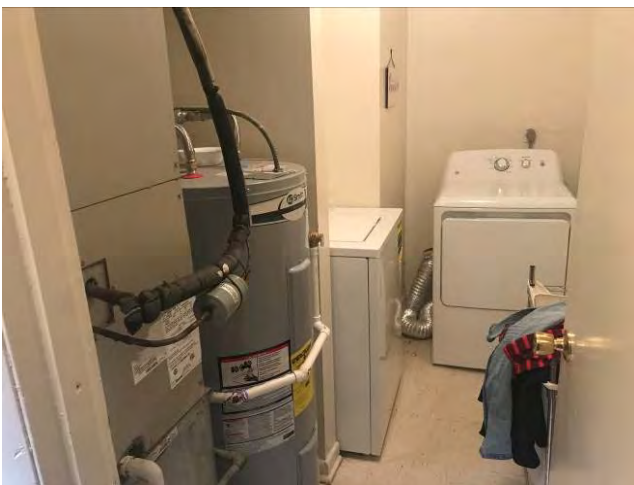
UTILITY CLOSET & W/D APPLIANCES
