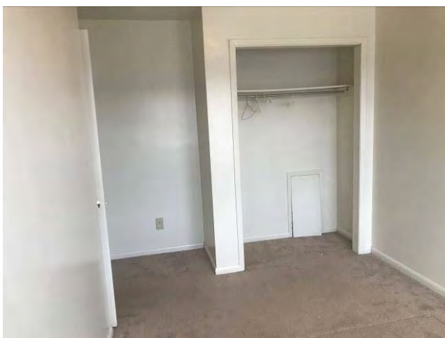
TYPICAL BEDROOM / CLOSET (VACANT 2BR)
