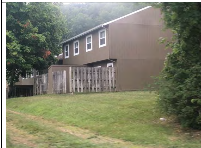
SUBJECT EXTERIOR AND FENCED PATIO
