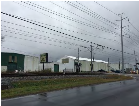
View of site facing southwest from Curlew Drive
