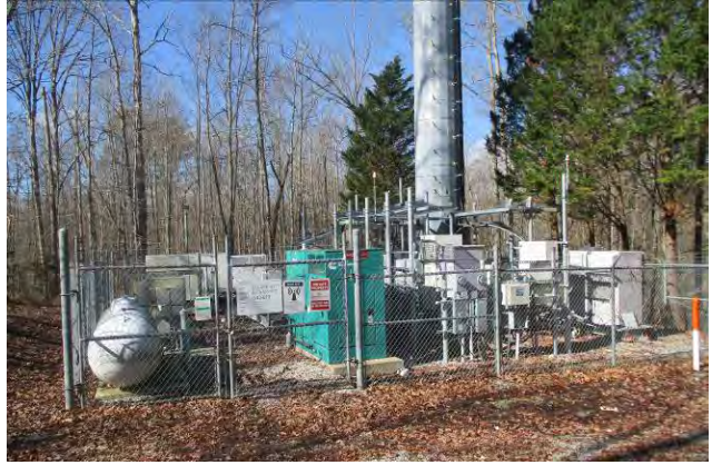
UTILITY USE SOUTH OF SUBJECT SITE
