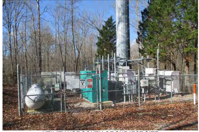
UTILITY USE SOUTH OF SUBJECT SITE
