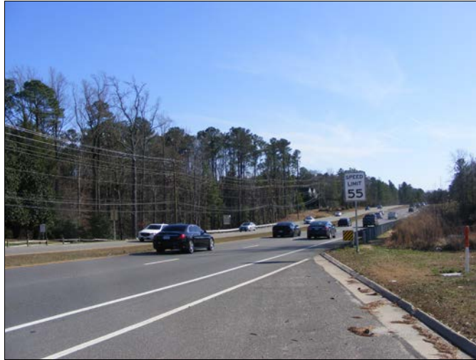
View south on Iron Bridge Road, at site
