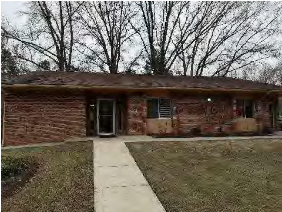
View of Accessory Building Exterior
