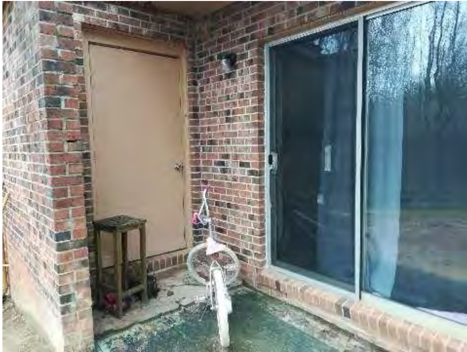
View of Typical Patio and Extra Storage
