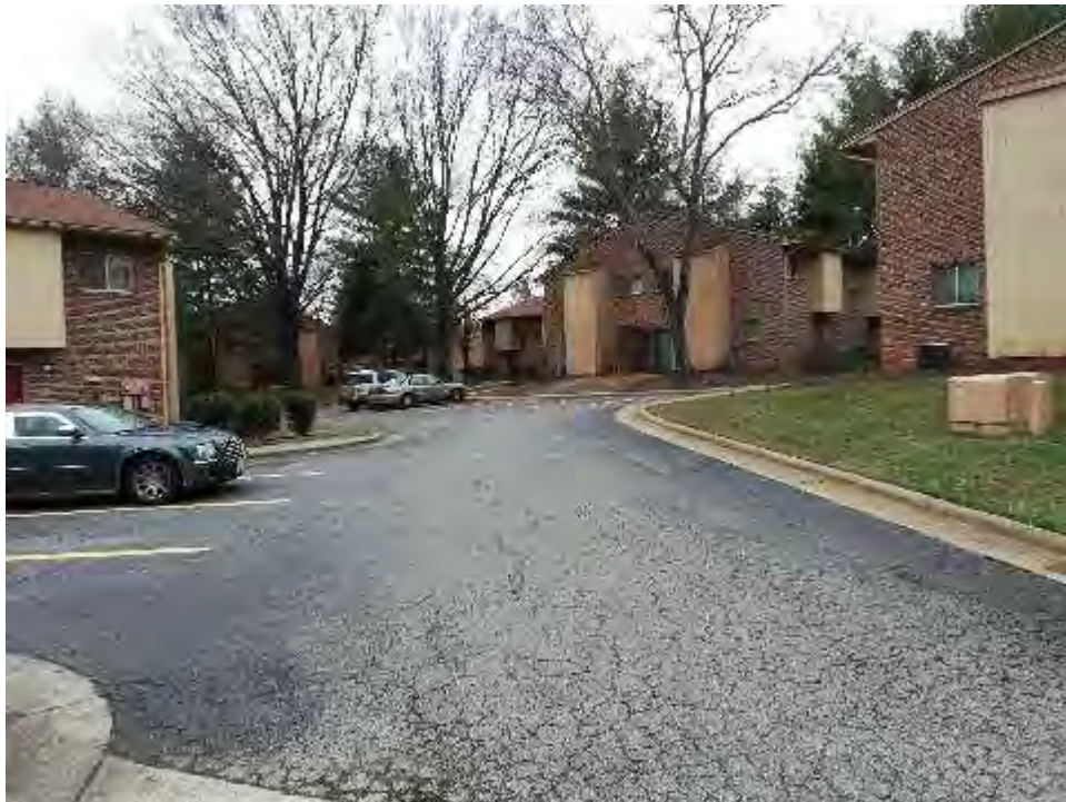
View of Parking
