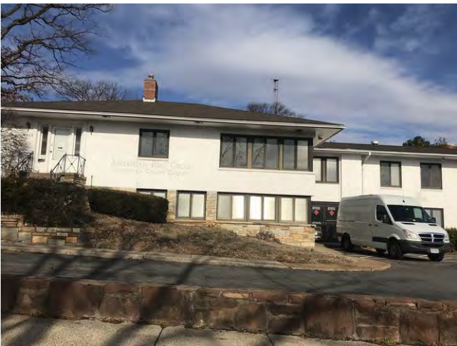
American Cross building directly southwest of the Subject to be demolished to make way for The Cadence, a new construction LIHTC property
