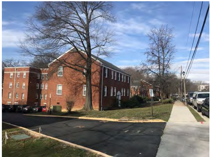
Subject exterior and parking lot entrance
