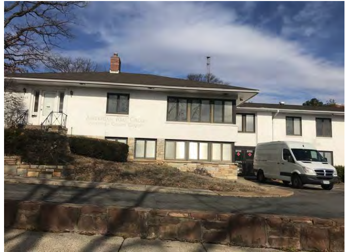
American Cross building directly southwest of the Subject to be demolished to make way for The Cadence, a new construction LIHTC property
