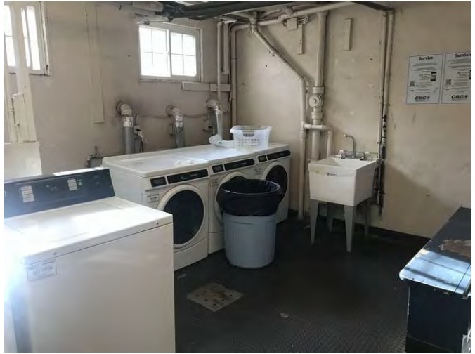
Subject central laundry facility
