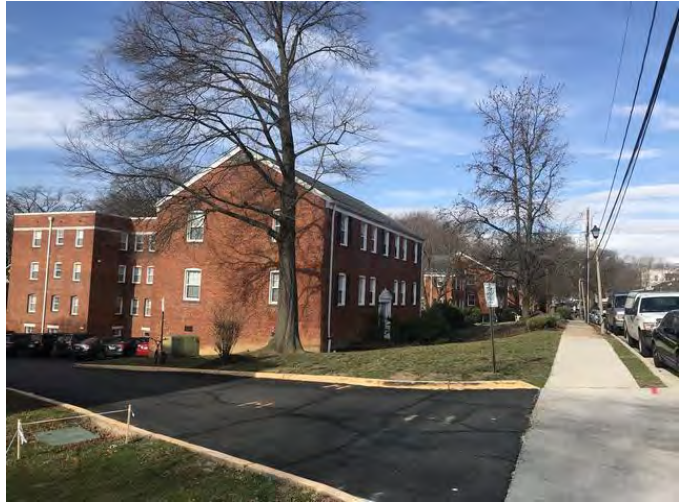
Subject exterior and parking lot entrance
