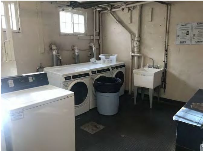
Subject central laundry facility
