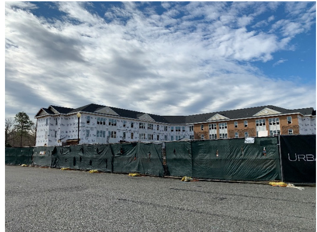
Market Square IV (Under Construction)
