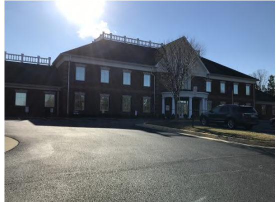
Office building southeast of site on Wylderose Drive
