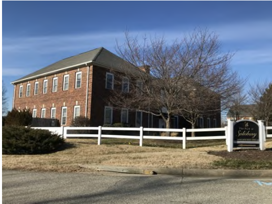
Typical office building, east of site on Wylderose Drive
