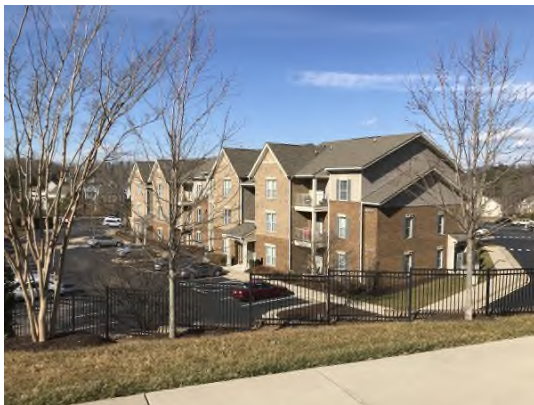
Brook Creek Crossing Apartments, north of site
