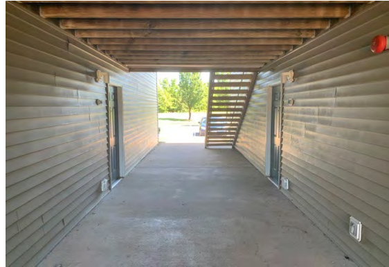
Exterior Corridor - Aspen Club
