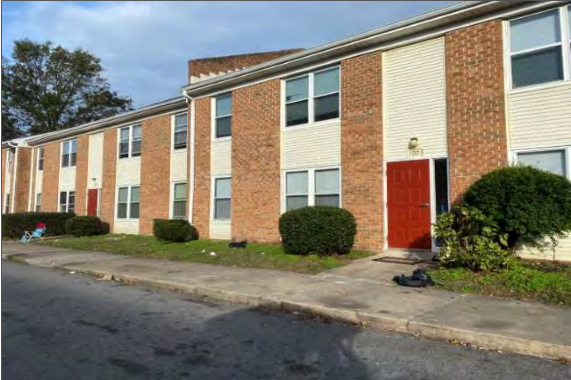
Exterior view of subject building
