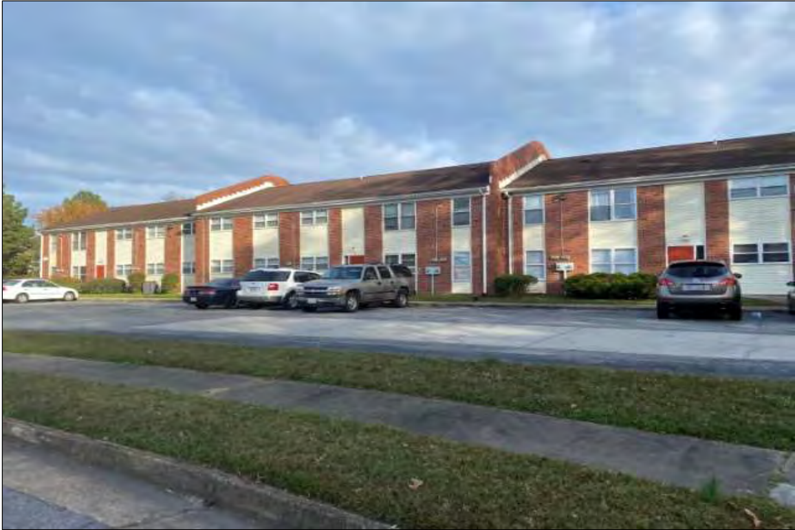
Exterior view of subject building
