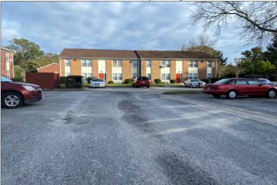
Exterior view of subject building
