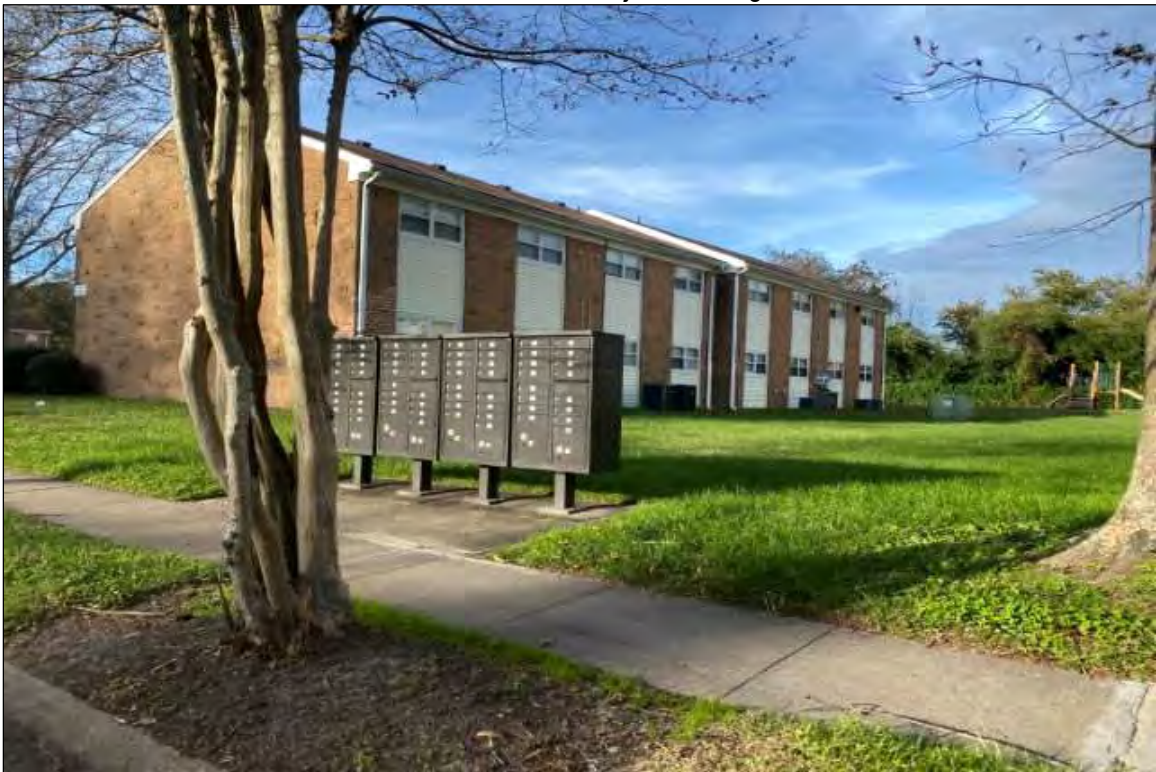
Exterior view of subject building and resident mailboxes
