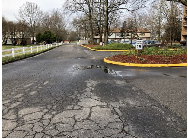
View along Old Iron Court facing west
