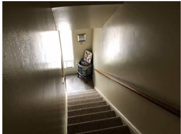
Typical in-unit stairway
