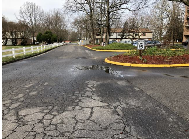
View along Old Iron Court facing west
