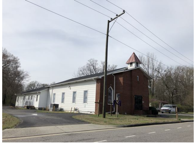
House of worship to the east of Subject along Courthouse Road
