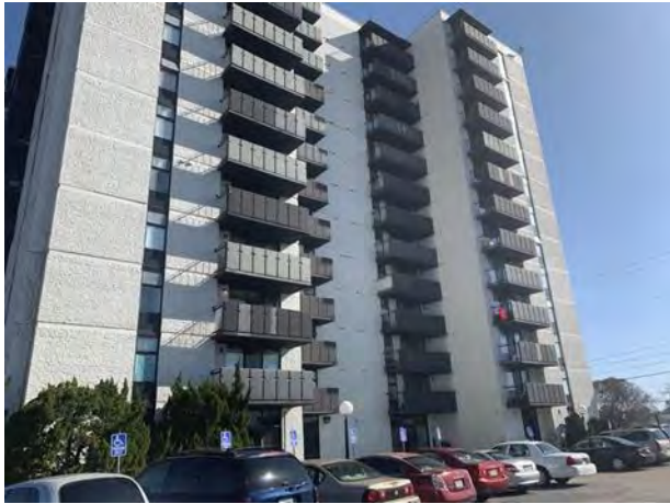
Subject building from entry drive
