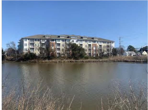
Alternative view from rear of Subject property
