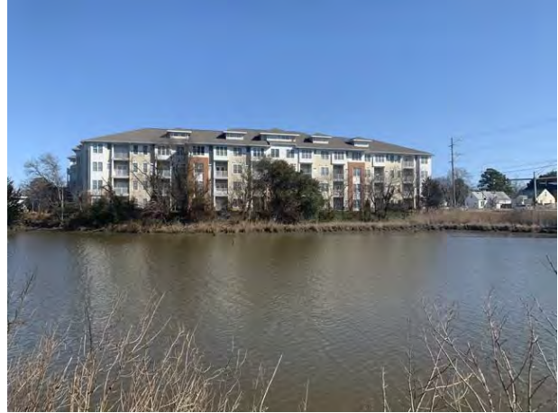
Alternative view from rear of Subject property
