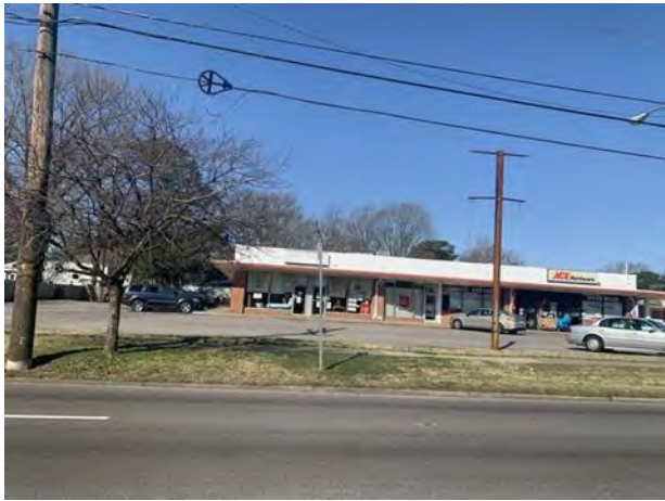
Strip center in average condition on Tidewater
