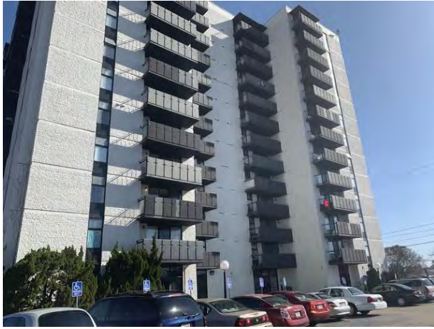
Subject building from entry drive
