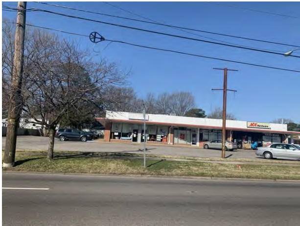
Strip center in average condition on Tidewater
