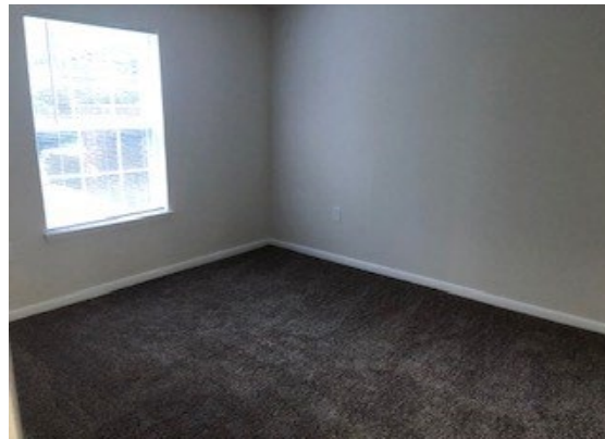
Typical Unit Interior
