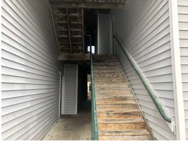
Typical exterior stairway
