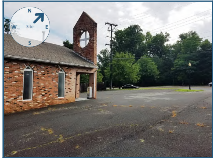
Northeast view from site
