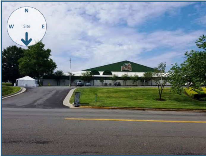
South view from site
