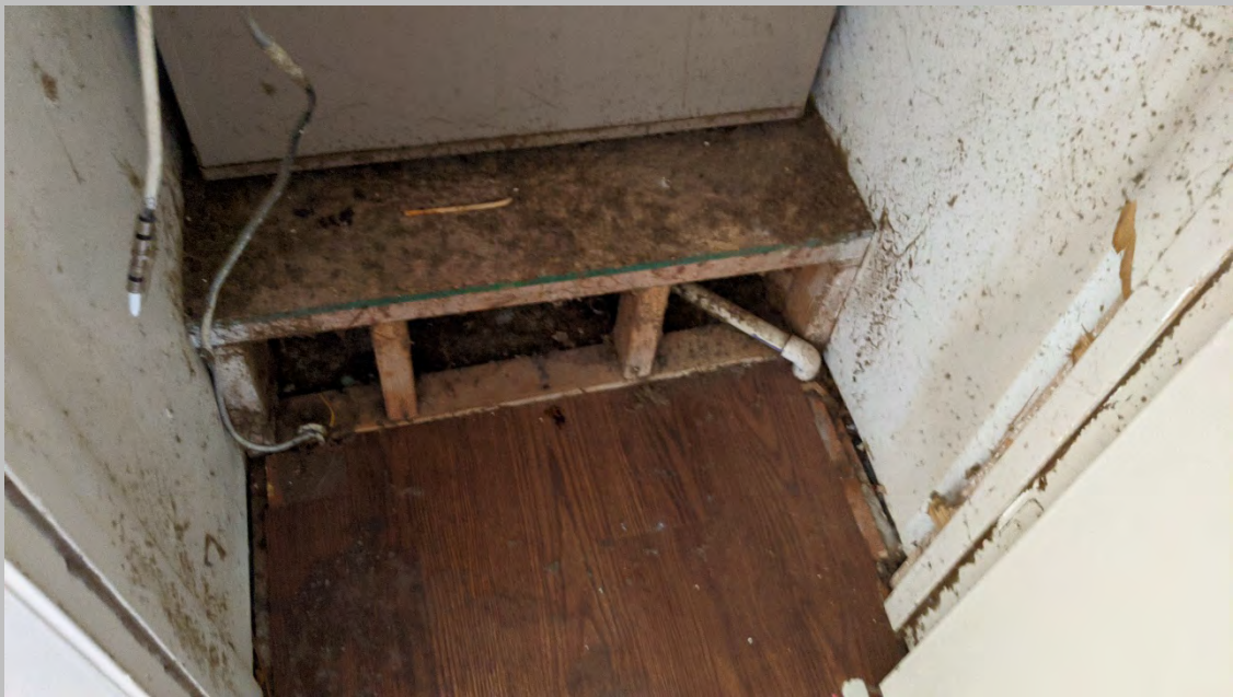
Typical Air Return Plenum for HVAC Units
