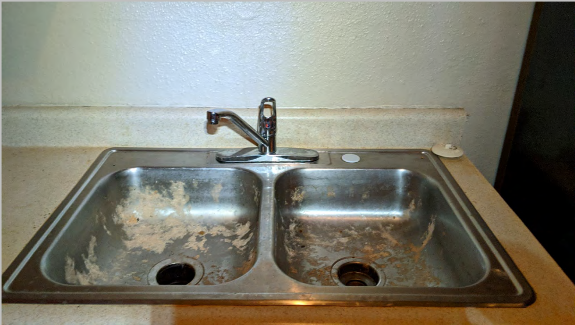
Typical Kitchen Sink
