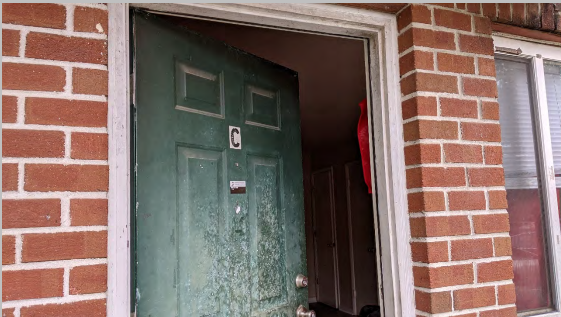
Entry Doors are Hollow Metal or Polystyrene
