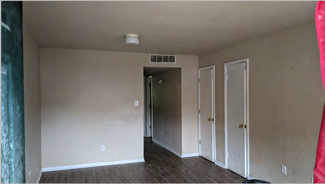
Soffit Containing Duct Work for Dwelling Units
