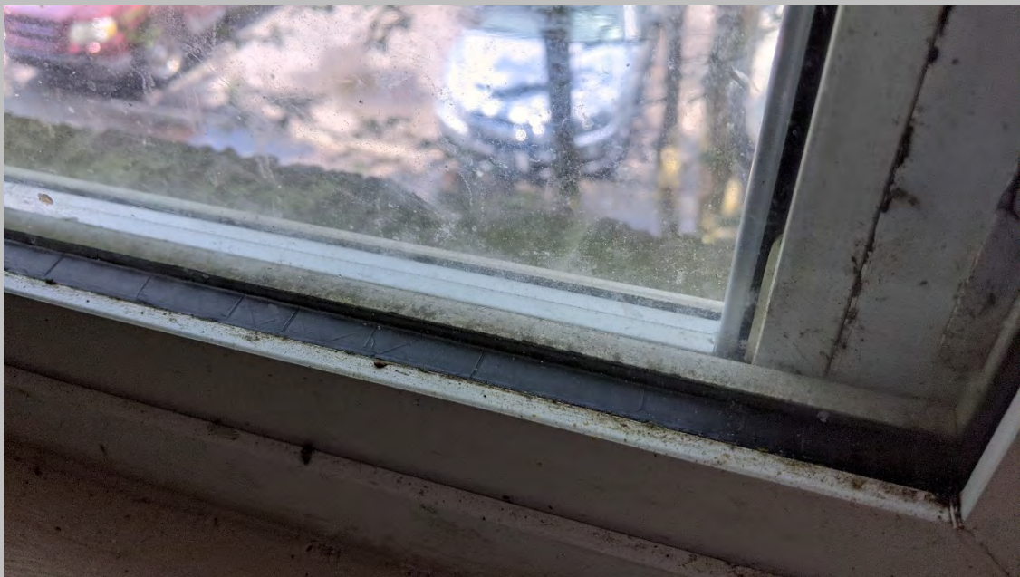
Typical Double Pane Clear Glass Window at Dwelling Units (close up view)
