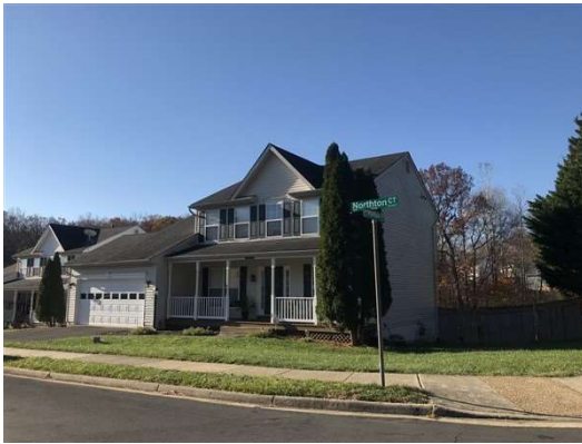
Single-family home south of site
