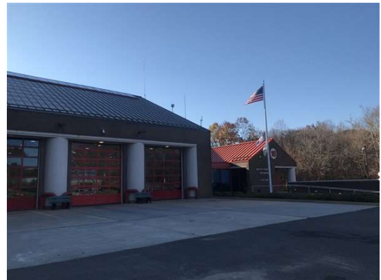
Fire station northwest of site
