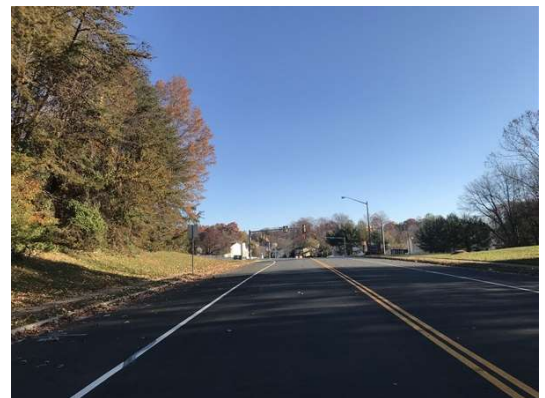
View of site southern boundary facing northeast along Princedale Drive
